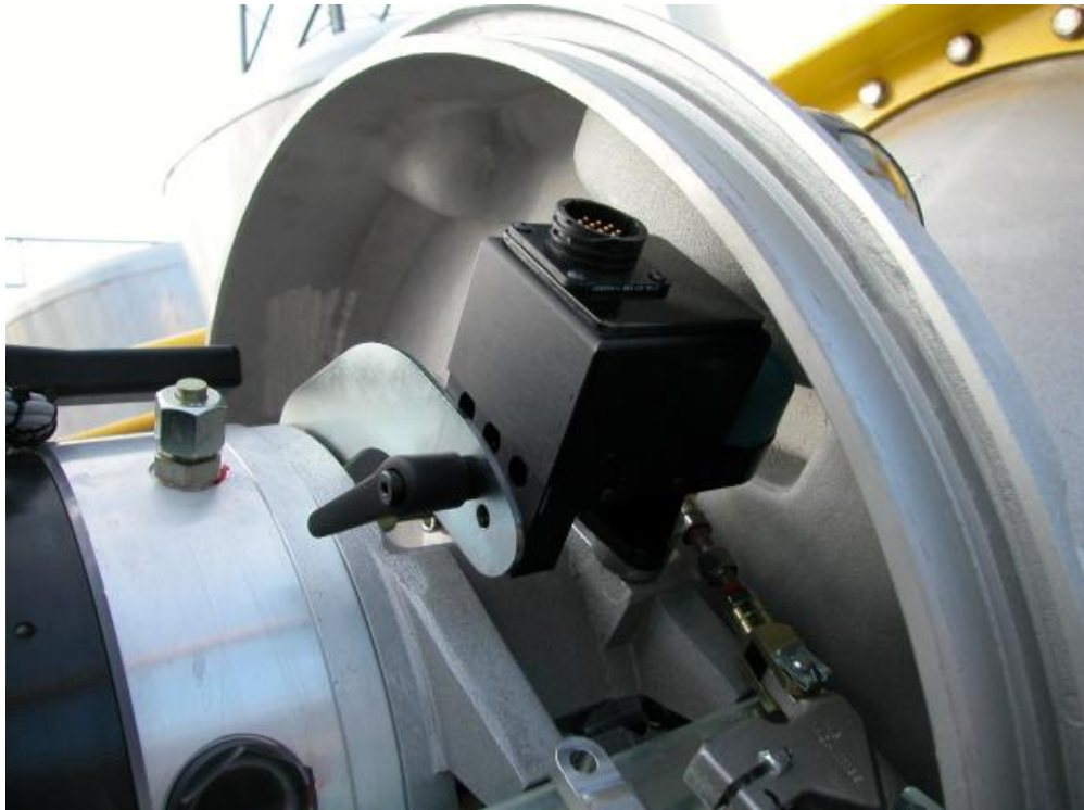
Rotary Transducer on ABB HMB Mechanism
